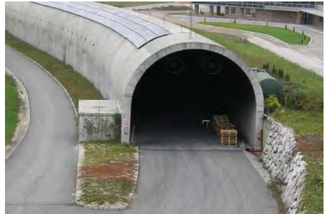
The full scale tunnel on the TST site in Spain dedicated to all kind of tunnel fire tests
