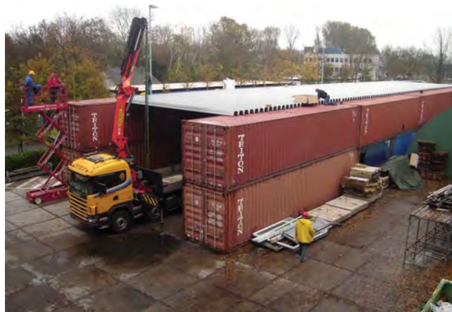
Construction of a temporary tunnel for ad-hoc fire testing
