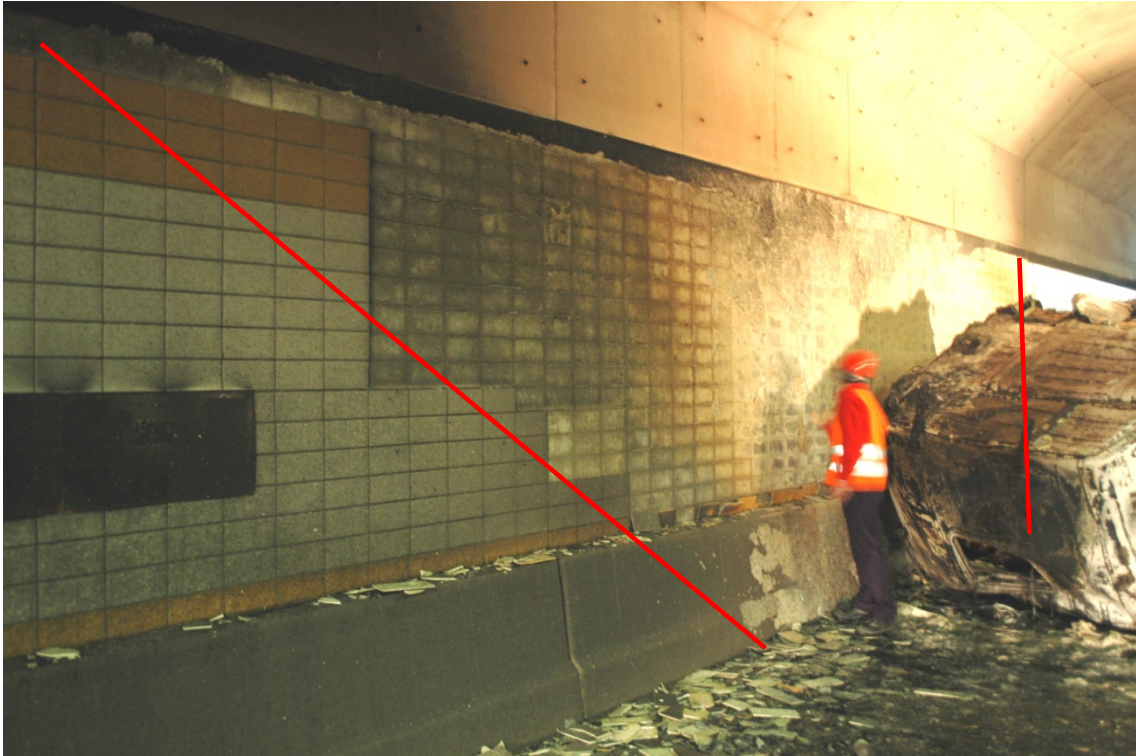
Figure 9 Damage pattern on the tunnel wall
