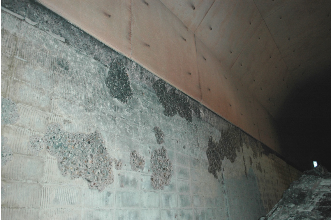
Figure 10 Spalling of concrete
