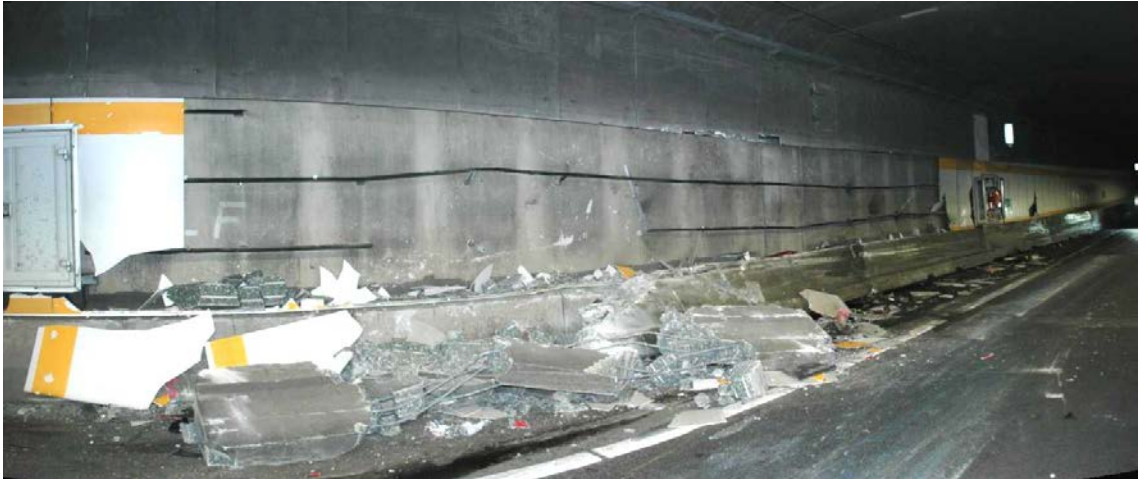
Figure 12 Damage to the barrier and the left tunnel wall due to the crash
