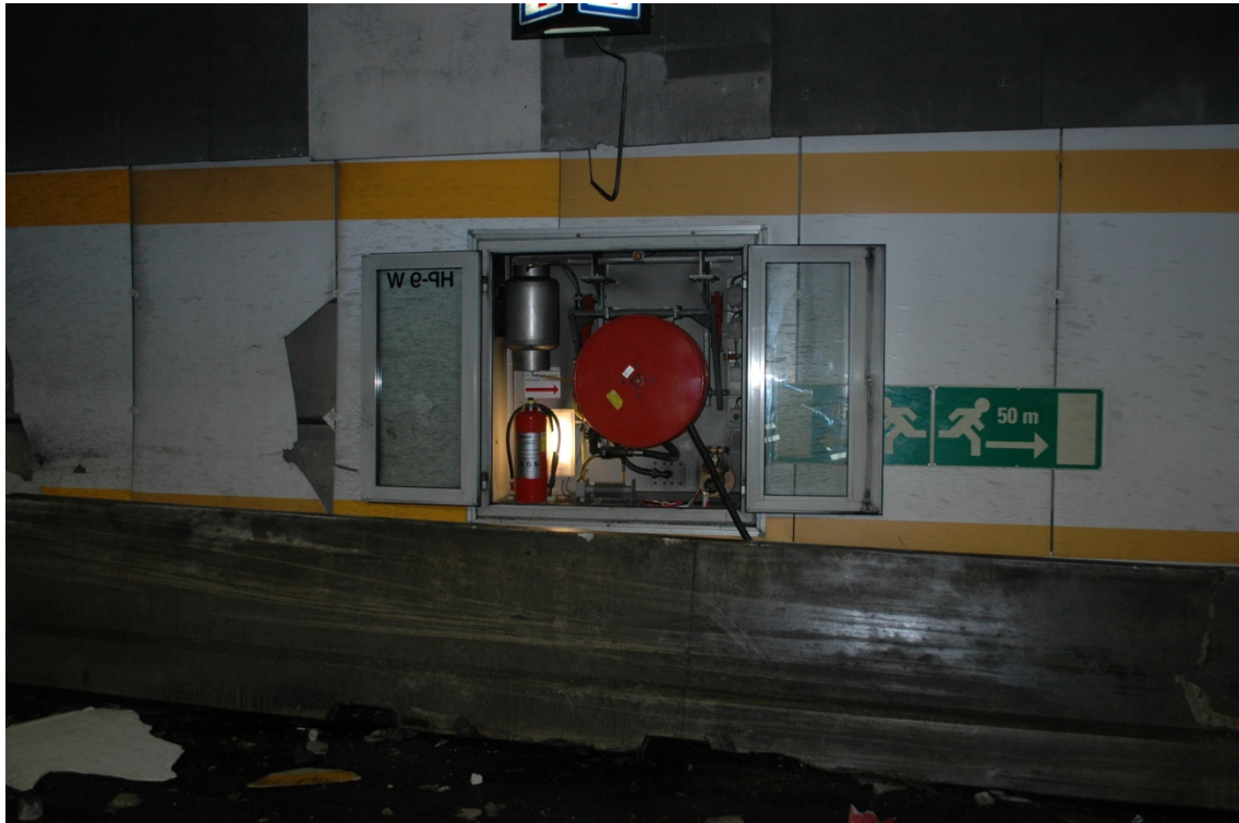
Figure 4 Fire fighting equipment and escape route signs
