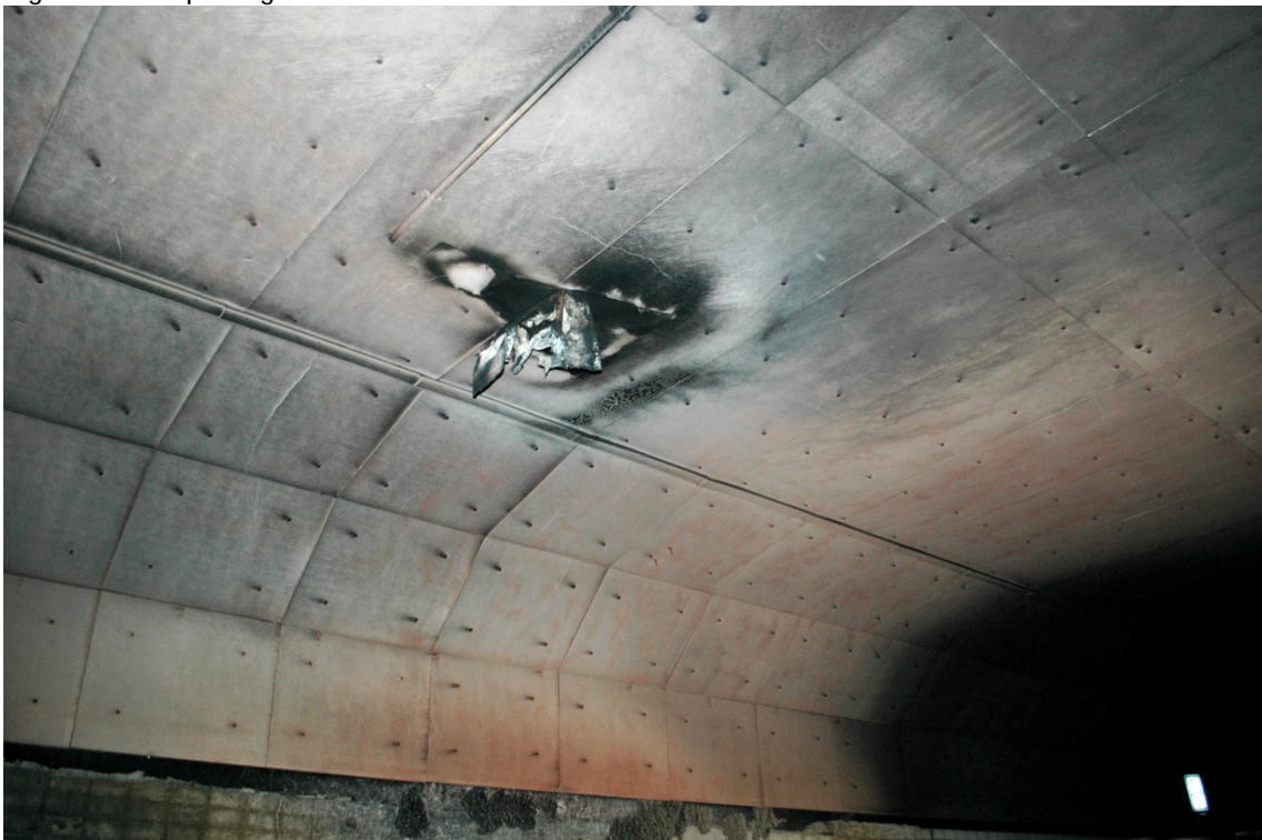
Figure 11 The tunnel lining directly over the cabin shows a clean burn.
