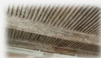
Diagnostic plancher bois
