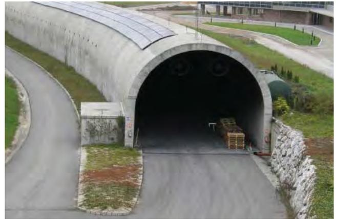
*The full scale tunnel on the TST site in Spain dedicated to all kind of tunnel fire tests*
